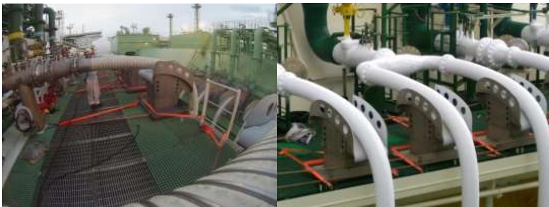
Figure 13–FSRU Saddles
