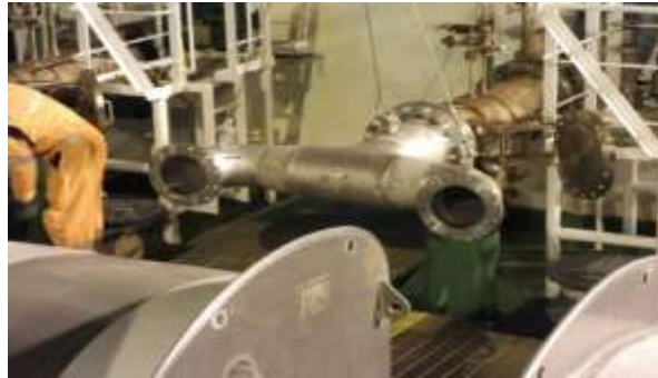
Figure 19: FSRU - Y Piece reducer
