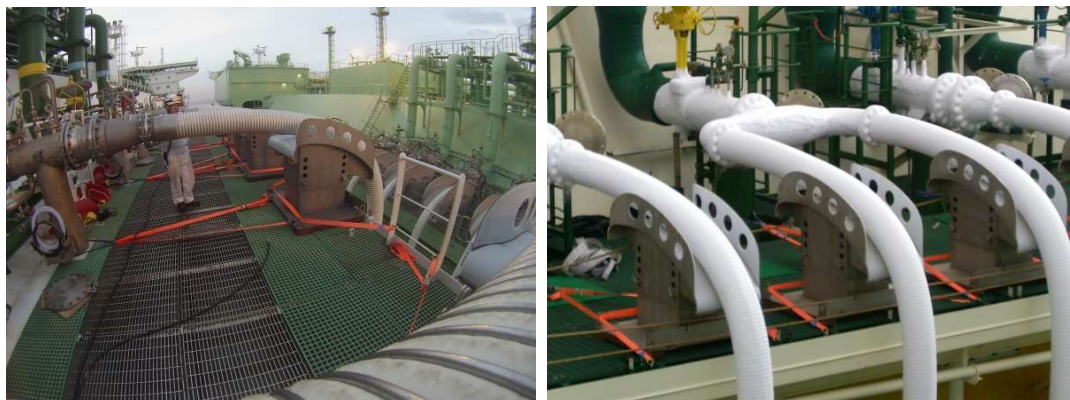
Figure 13 – FSRU Saddles
