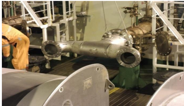
Figure 19: FSRU - Y Piece reducer
