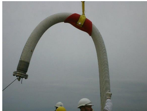
Figure 20: FSRU - Lifting with hose bun
