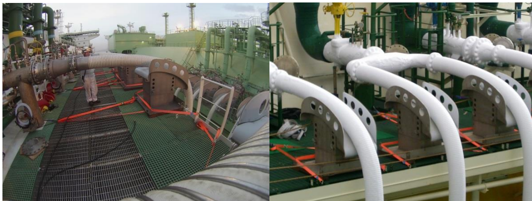
Figure 13–FSRU Saddles
